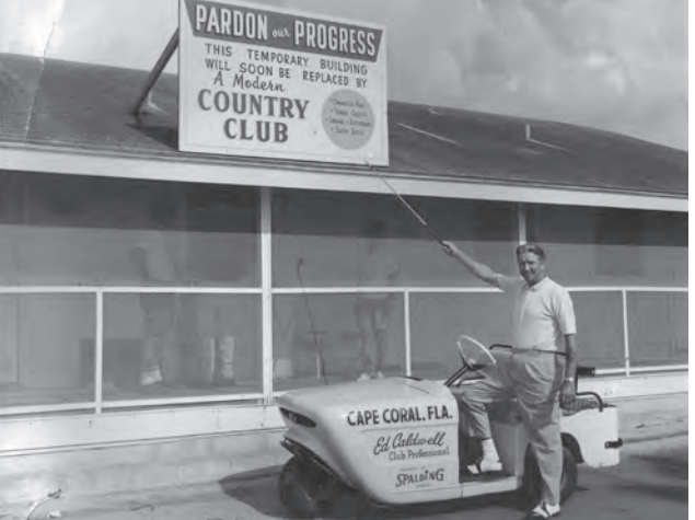
Cape Coral Country Club golf course opened to the public on July 8, 1961, with a nine-hole golf course, and a second nine holes opening the following year. The building shown was originally used as the pro shop and snack bar and now serves as the offices and museum store for the Cape Coral Museum of History. The Cape Coral Country Club closed in 2006.
