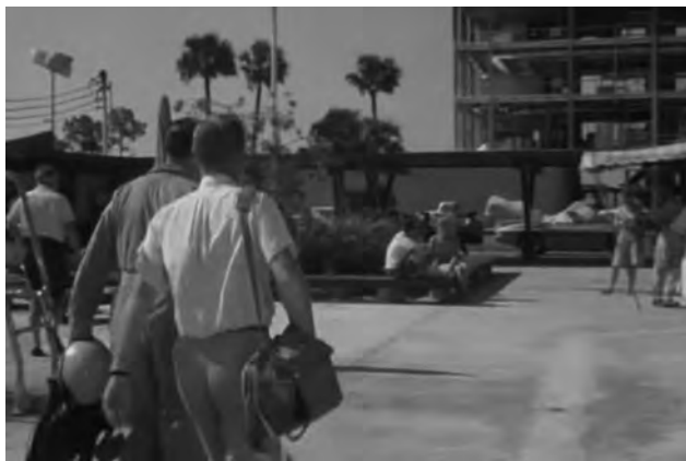
A photo from the Route 66 Two Strangers and an Old Enemy episode with the Gulf American Land Corporation building being built in the background. Located at: 4732 Del Prado Blvd. S.
