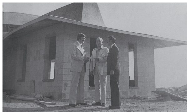
The Chamber of Commerce of Cape Coral building was constructed in 1977.
